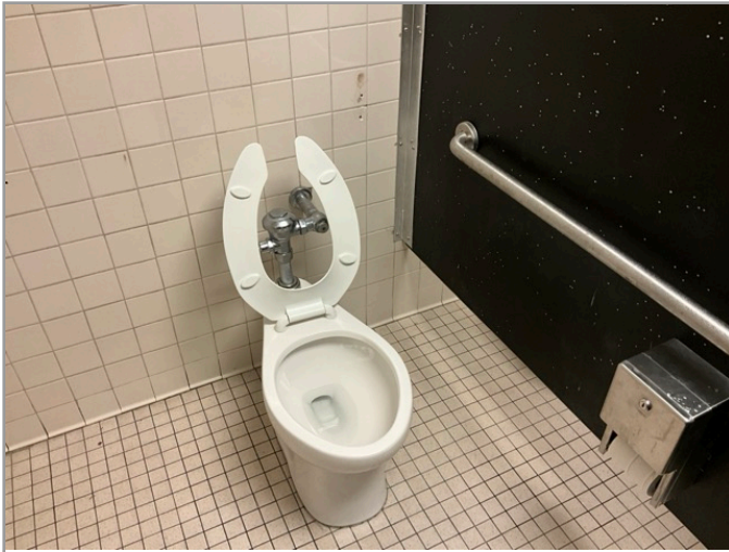
TOILET STALL OVERVIEW
