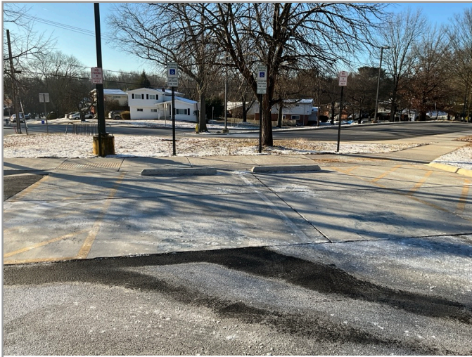
OVERVIEW OF ACCESSIBLE PARKING AREA
