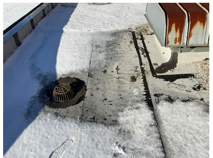
6 - PRIMARY ROOF OVERVIEW
