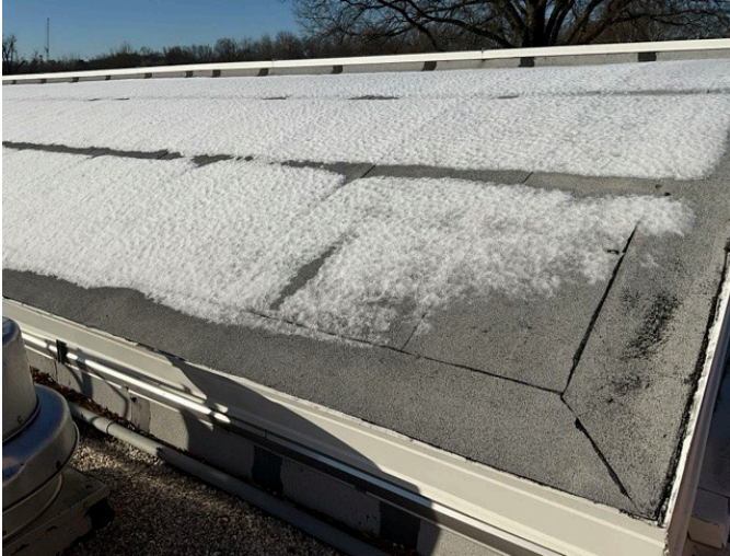
7 - PRIMARY ROOF OVERVIEW
